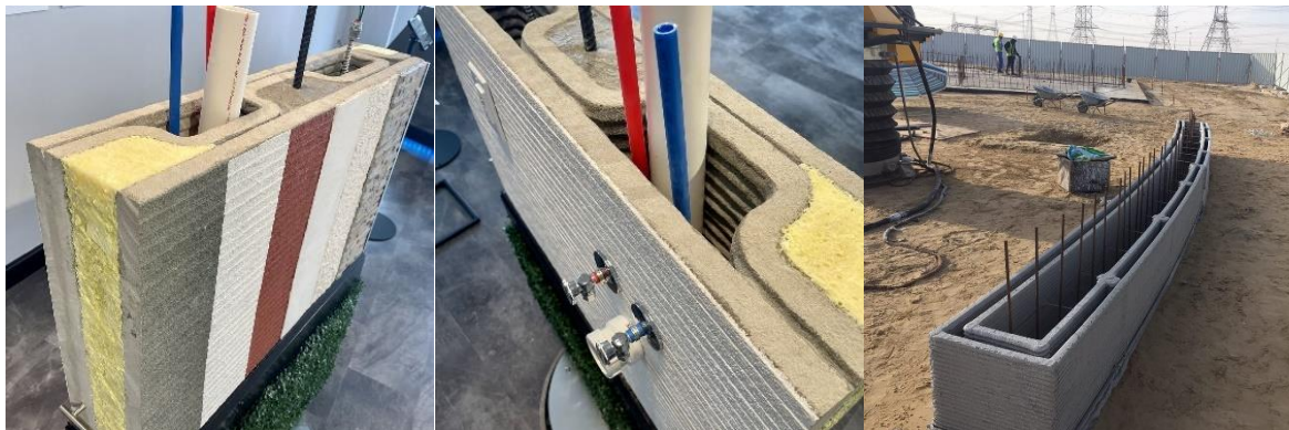
Fig. 3. Details of a 3D printed wall by Apis Cor [6]
